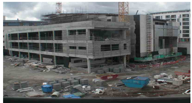
Building work progress at PRONI Site September 2009.
