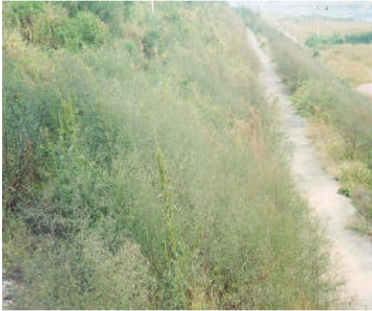
Figure 7 Embankment with soil covering and vegetation
