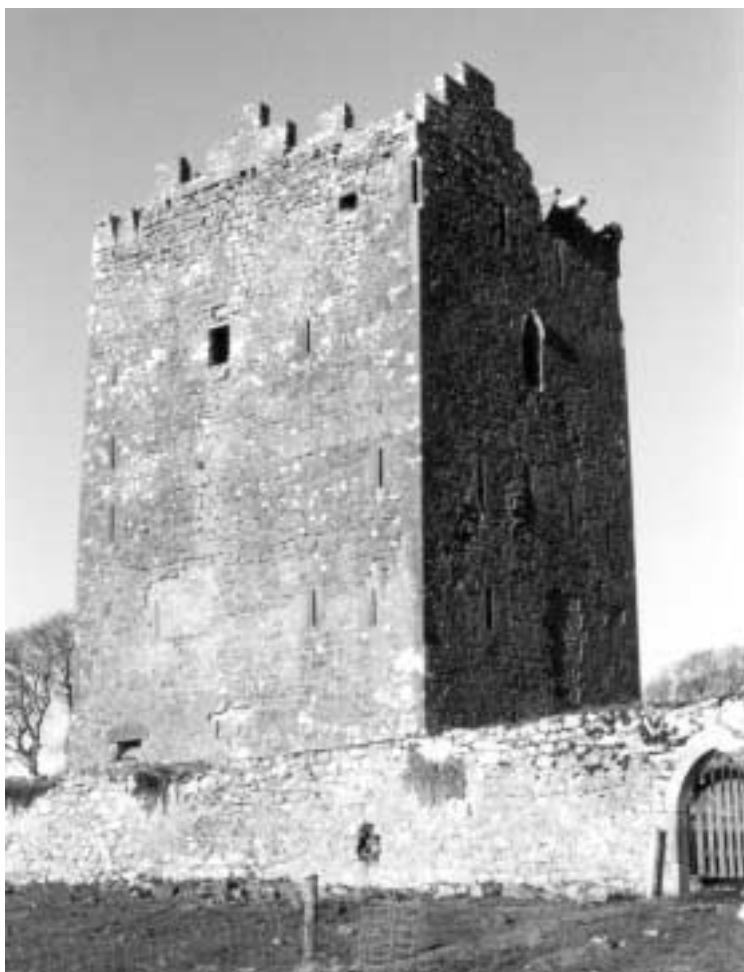
Figure 6: Lackeen Castle, county Tipperary, an early sixteenth-century tower-house of the O'Kennedy family.
