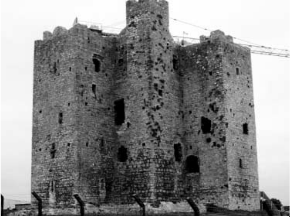
Figure 4: The donjon of Trim Castle, county Meath, during recent conservation work.
