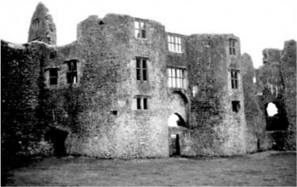
Figure 1: Roscommon Castle. The towers and adjoining walls of this castle were erected shortly before 1300, and new windows were inserted in the late 1500s. The centuries between these dates, as well as the period after 1600, are not discussed in the archaeological literature.
