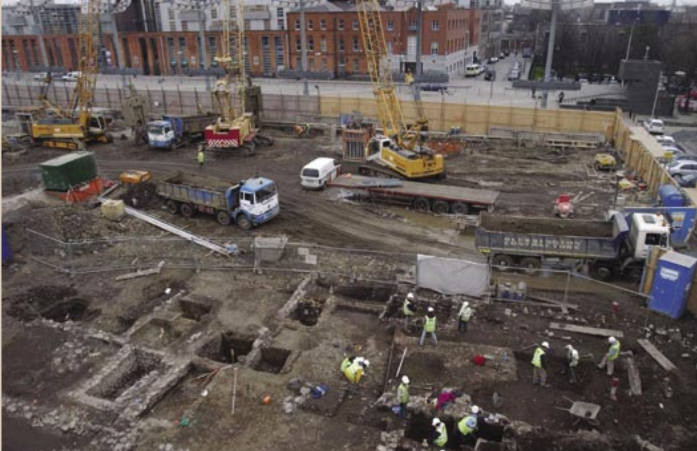
Excavation of 17th and 18th century structures at Smithfield, Dublin. Excavation was undertaken in two phases to facilitate construction. The well-preserved remains were of buildings and properties shown on John Roque's map of Dublin in 1756 [Margaret Gowen and Co. Ltd]
