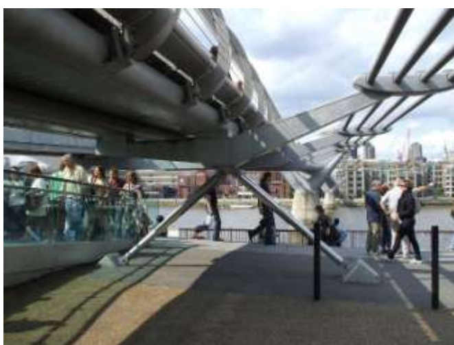
1. Millennium Bridge, London and its ‘fluid dampers’ 14
