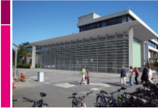
Computer generated image of the new UCD Research Centre
