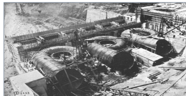
1925 Shannon hydro-electric scheme, Ardnacrusha
