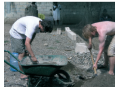
Conal Ryan & Paul Healy, final year Architecture students at work renovating the local poorhouse
