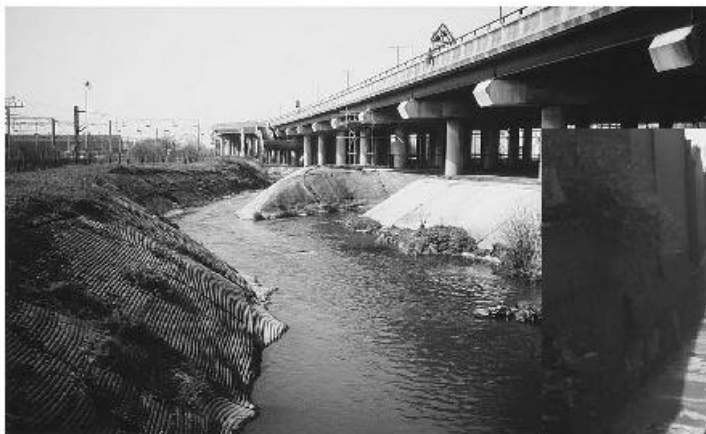
River Tame under the M6 motorway
