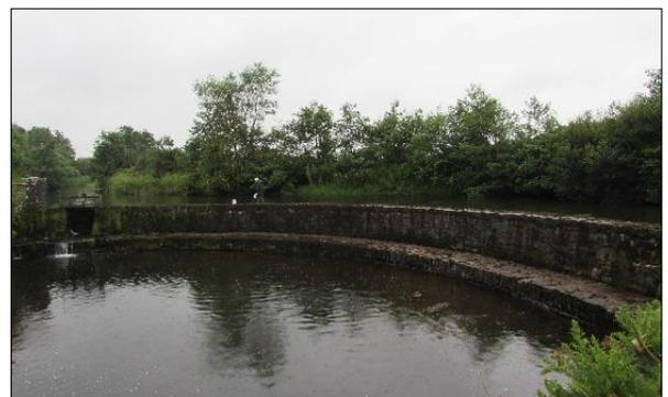
**Historical 25" map** drawing of a weir on the Nore (photograph on the right) known as "The Basin". This weir was constructed in the late 1800s. Like many fish passes built at that time, the pass shown in this map is specifically designed for salmon and may not work for other native species (e.g eel, river lamprey, sea lamprey and cyprinids).
