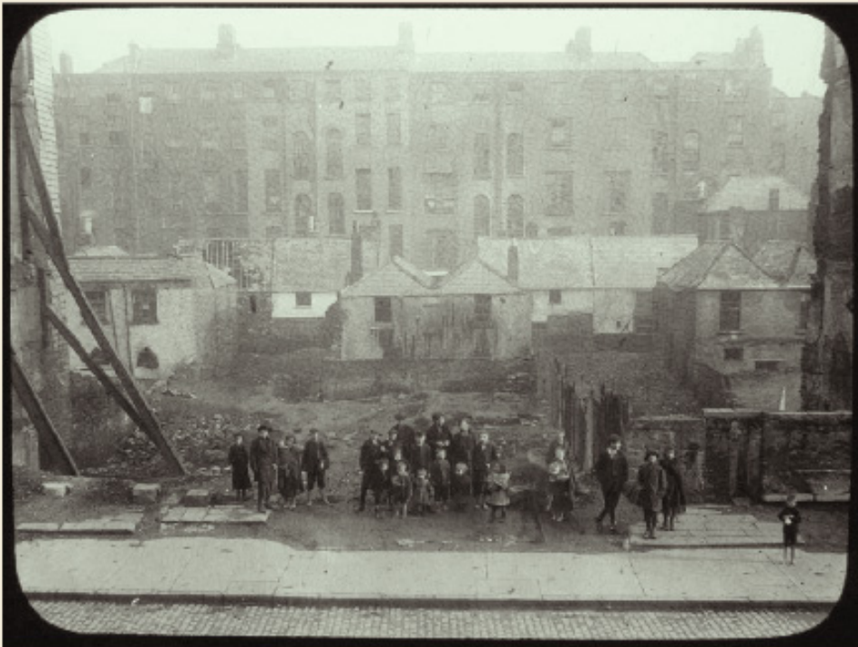
Fig. 1. Tyrone Street, backing onto North Cumberland Street, in 1913 (RSAI, 'Darkest Dublin' Collection). Reproduced by permission of the Royal Society of Antiquaries of Ireland ©.
